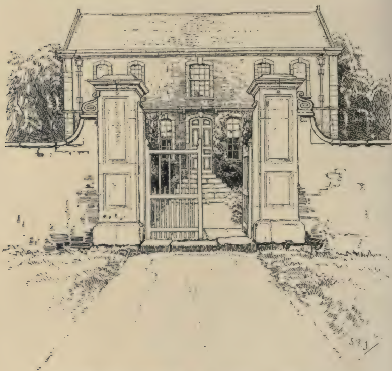
THE MANOR-HOUSE AT ATWORTH, WILTSHIRE
